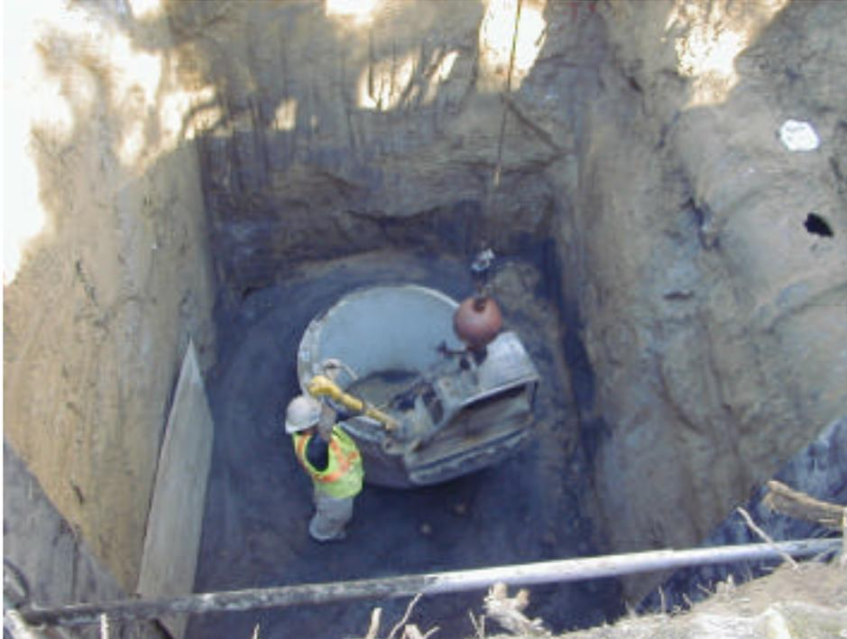
Workers lower a section of the new storm drain filter into an 18 foot hole at Bellevue and Staten by outfall # 4. First of the measure DD projects, it will remove trash from 26 acres of Grand Avenue and nearby streets. The 24 inch storm drain to which it will connect is on the right.
