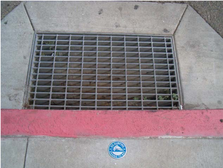
View of storm drain marker adjacent to storm drain
