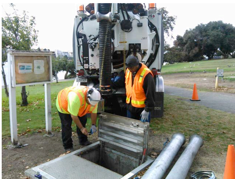
City staff inspect - clean a storm drain filter near the Lake
