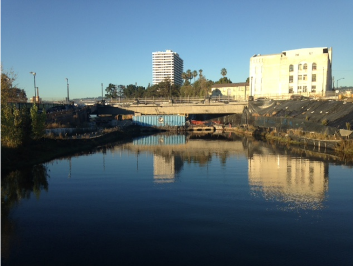
The Lake Merritt Channel at 10th St. (under construction)
