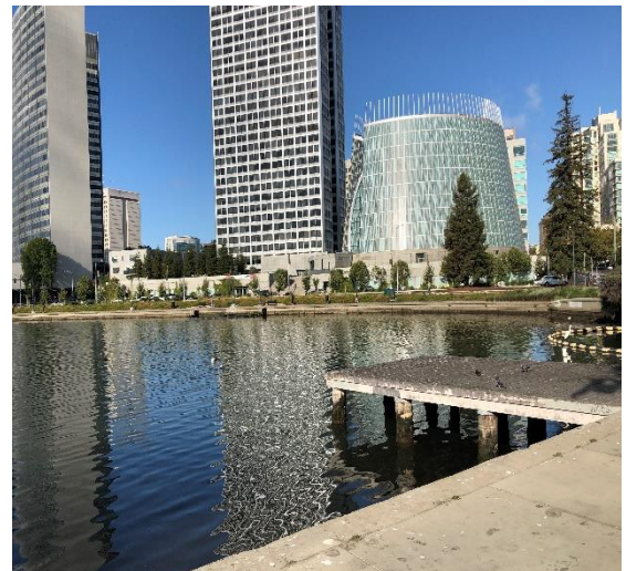
Fountain Missing at Glen Echo Inlet
