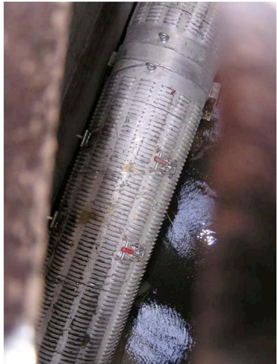
*A continuous, in-line, storm drain detention device, recently installed at the 12<sup>th</sup> Street project.*
